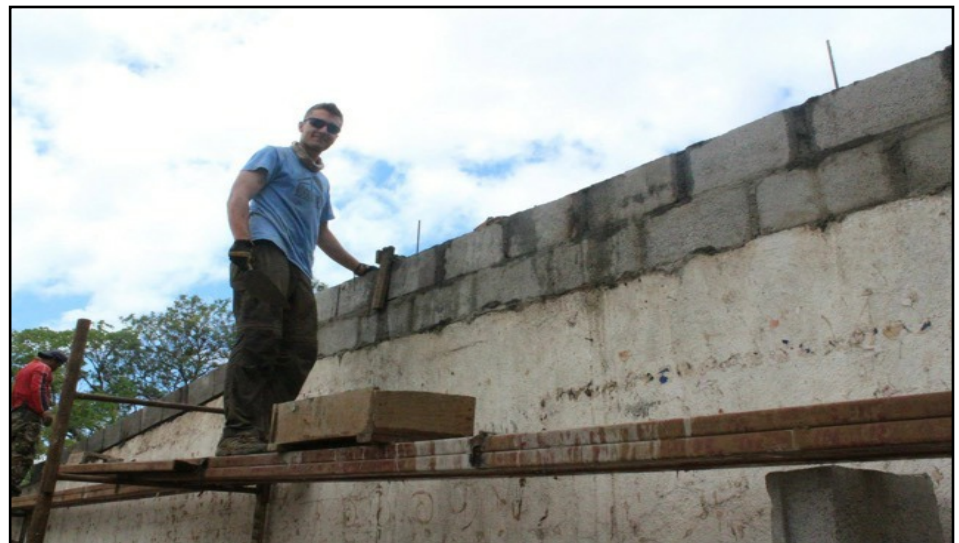
Above, Brennon Thompson adds height to the auditorium walls.
